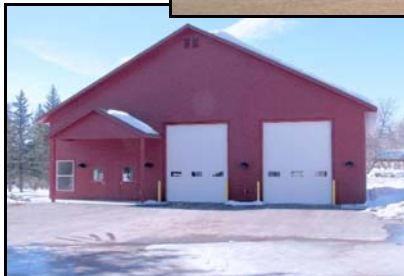
Alton Town Fire Station
