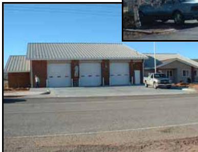
Hurricane City Fire Station Brentwood Area
