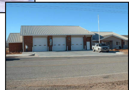
Hurricane City Fire Station Brentwood Area
